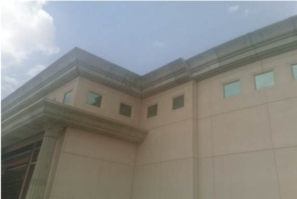
Project Name : Jareer Boock store Customer Name : Arabian Services Contracting Co.
