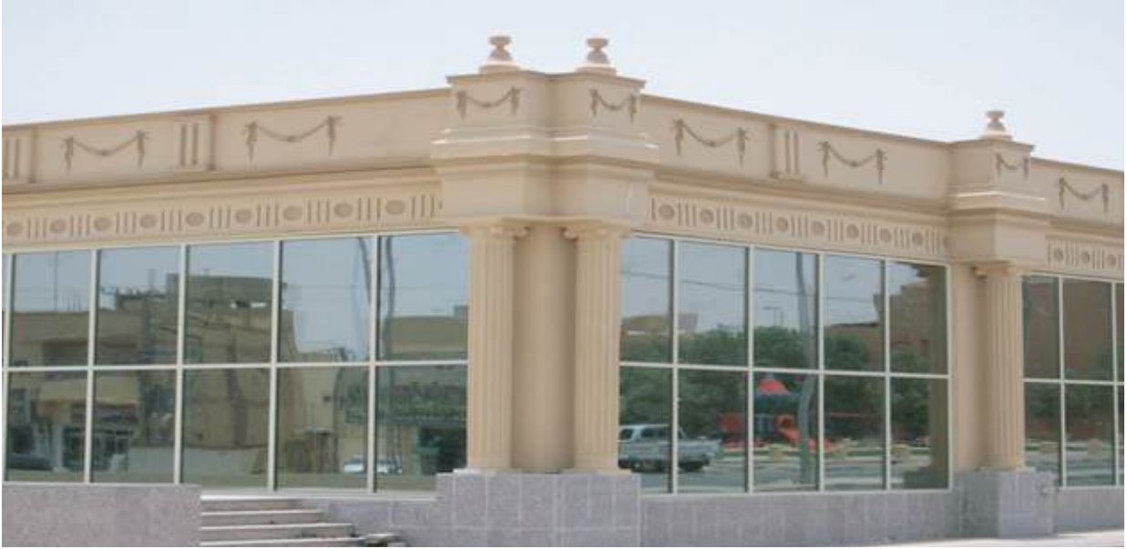
Project Name : Al-Muzahmia Mall . Customer Name : Aba Namy Contracting Co
