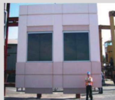
Panel assembly prepared for installation
