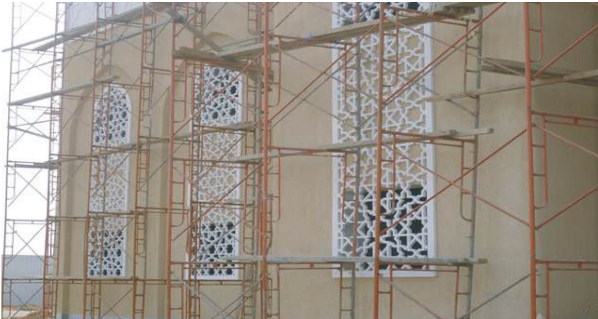
Project Name : Court Building . Customer Name : Al-Yamy Contracting Co.
